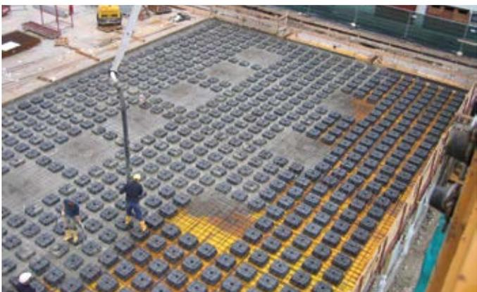
Figure 58 - casting of the first layer
