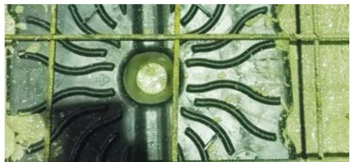
Figure 55 - cone correctly filled
