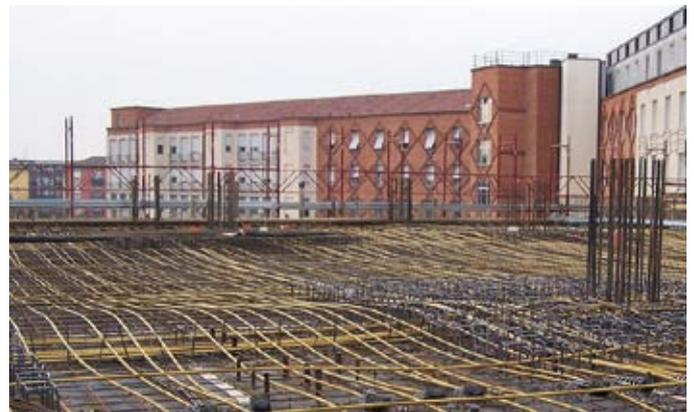
Figure 64 - post-tension cables on plate slab
