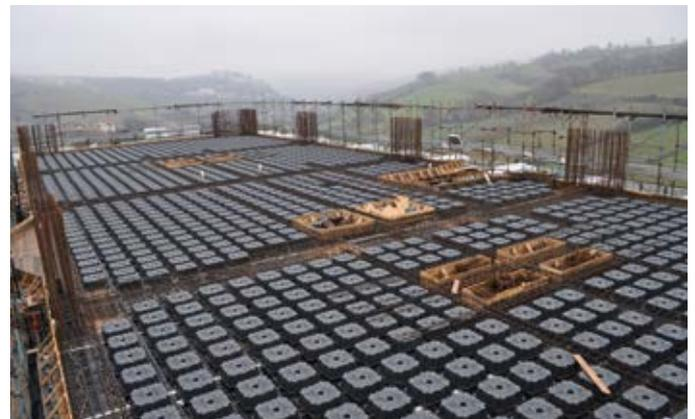
Figure 59 - preparation of cavities before casting
