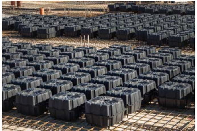
Figura 3 - layout of lightening New Nautilus Evo double
