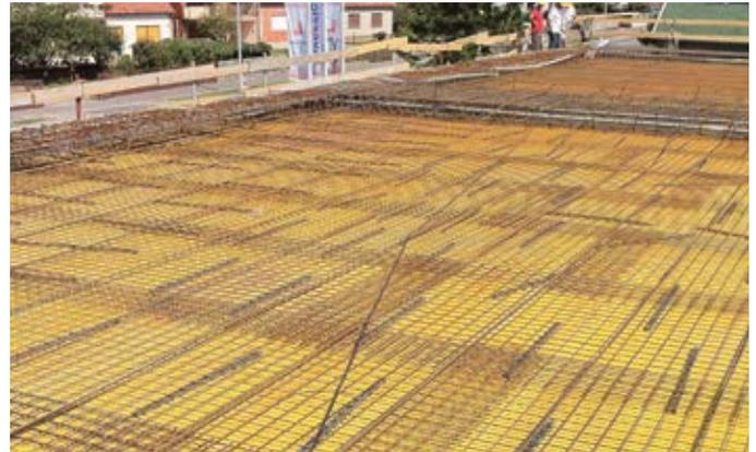
Figure 41 - laying of the lower reinforcement mesh
