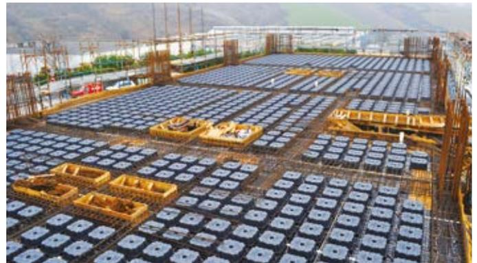
Figura 1 - lightened slab with New Nautilus Evo of Geoplast.
