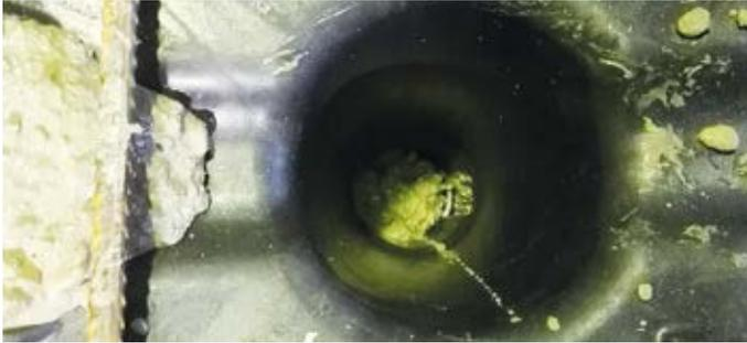
Figure 56 - cone not correctly filled, insist on vibration until reaching the situation of the previous figure
