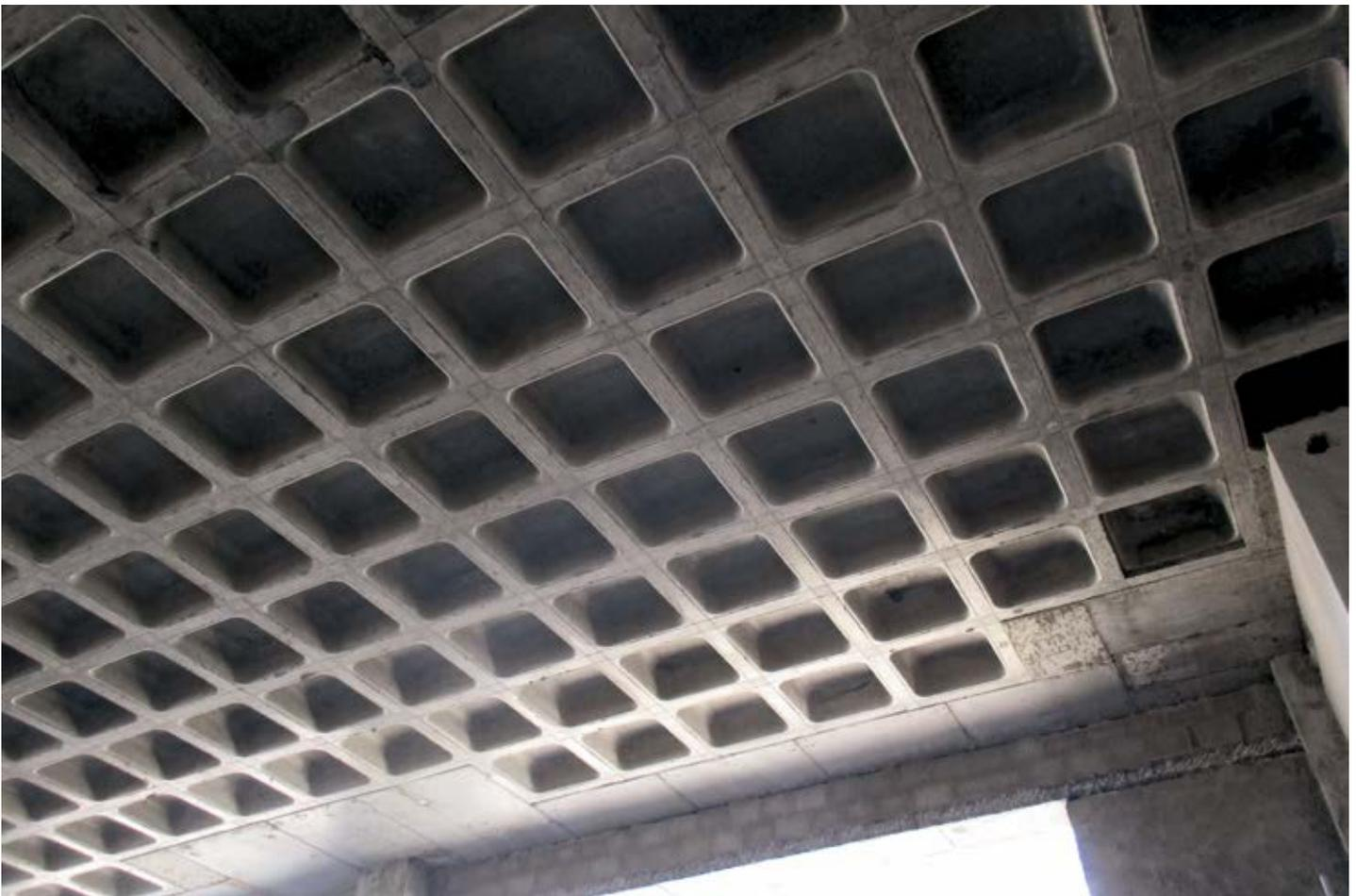
Figure 2 - example of reticular slab
