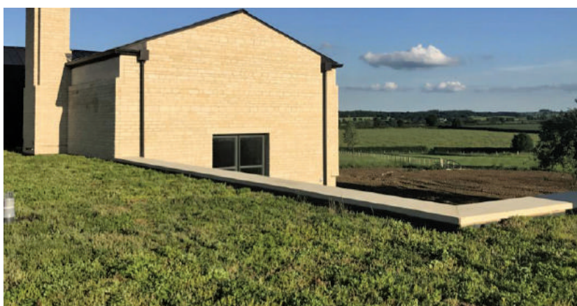
COMPLETA, 200 m 2 Micklands Hill Residence READING, UK
