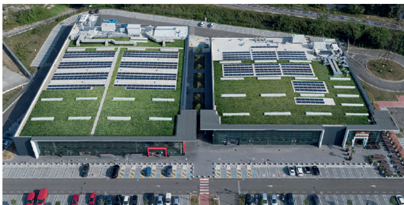
COMPLETA, 3200 m 2 SUPERMARKET BOLOGNA, ITALY
