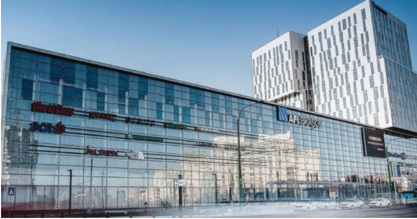
MULTIMODULO Centre commercial AFI BRASOV, ROUMANIE
